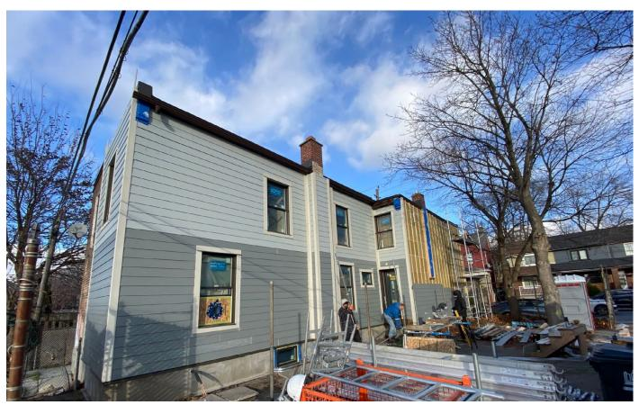
Building Up crew installs exterior insulation and cladding as part of retrifit project at NLT property at 262 Old Weston, 2023.
