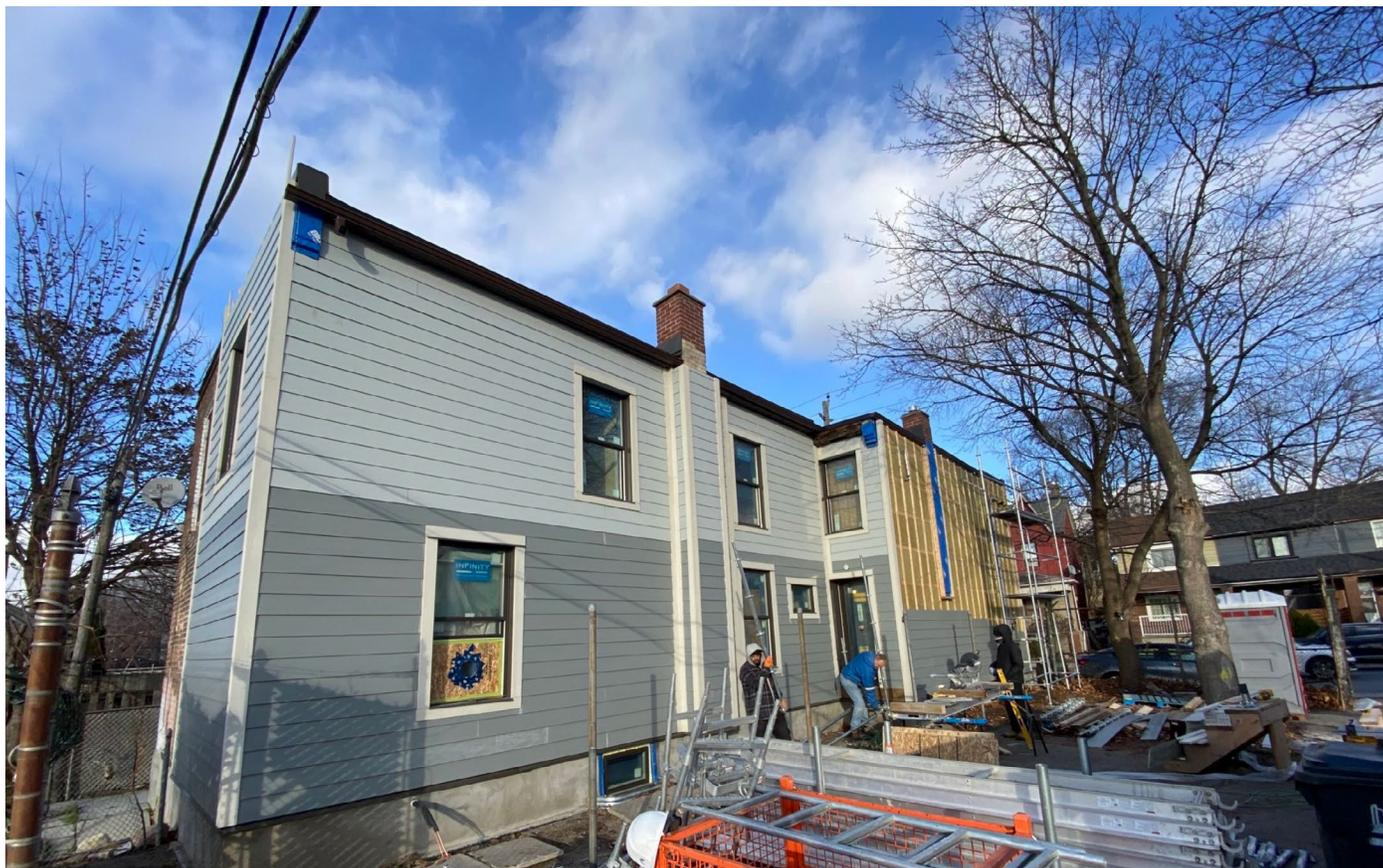
Building Up crew installs exterior insulation and cladding as part of retrofit project at NLT property at 262 Old Weston, 2023.
